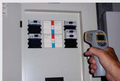
Find failed circuit breakers
